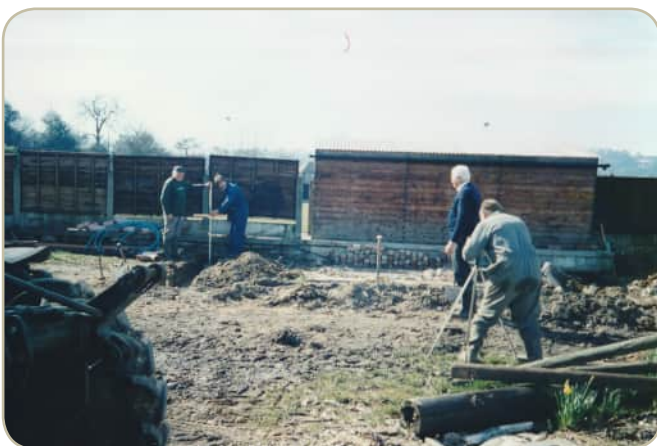
New pavilion build - 1995
